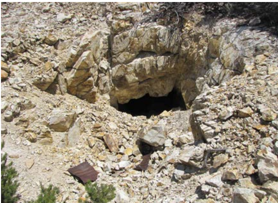
Photo 6. Example of mine hazards on BLM along SPOS boundary
